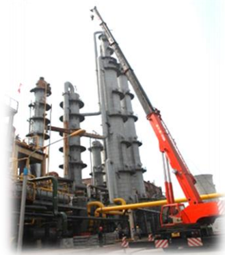
Reform of Gas Purification and Desulfurization System in Sinochem Changshan
